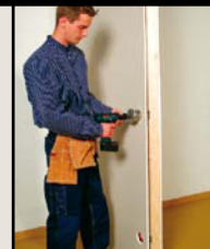
Drill a hole with a hole saw. Set the drill bit out as far as possible.
