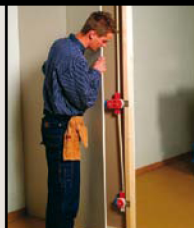
Mount the plaster-board/panel.
